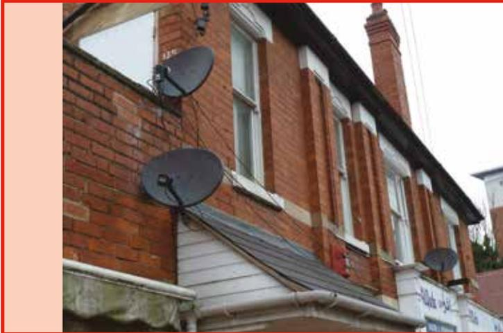
**POOR DESIGN.** Three poorly located satellite dishes on a single property, any redundant dishes should be removed and the rest should be relocated to the rear elevation away from the street.
