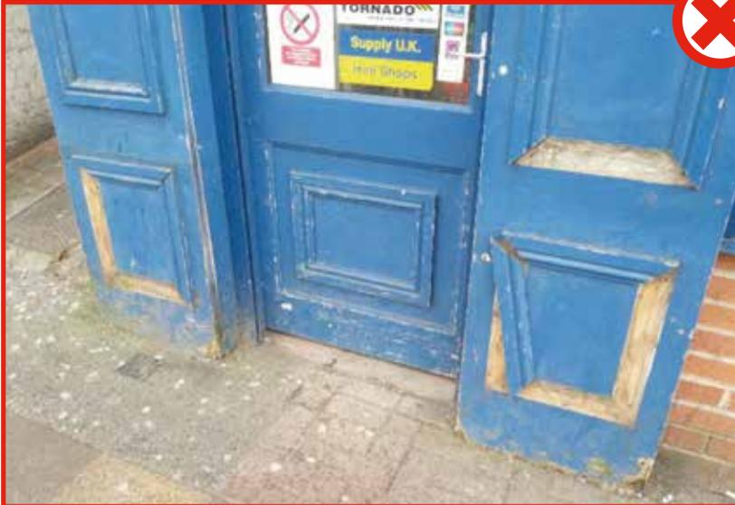
**POOR DESIGN.** Tacked-on moulding has been used to create decorative panels on this shopfront but they are poor quality, vulnerable to damage and quickly look tatty. Proper joinery techniques need to be used on timber shopfronts if they are to be robust and attractive.
