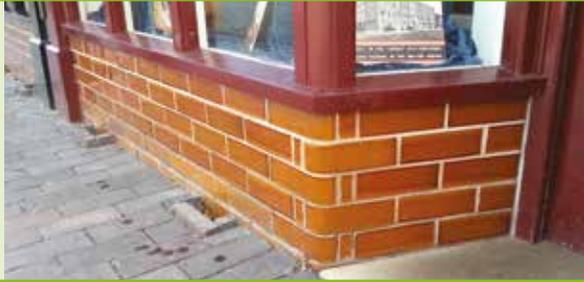
A glazed brick stallriser with a wooden cill above. Glazed bricks are easy to source and provide a robust and attractive shopfront feature.
