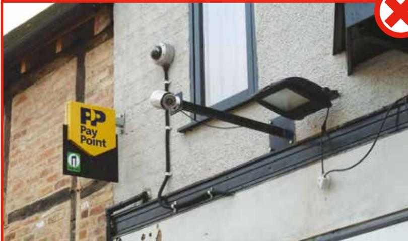
**POOR DESIGN.** Poorly located CCTV cameras with prominent wiring on a front elevation, it is unlikely that both are necessary in this location and one should be removed.
