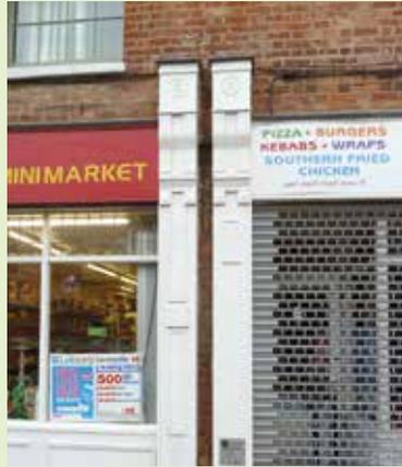
**GOOD DESIGN.** An open security shutter with the shutter box hidden behind the fascia and the side runners hidden inside the pilaster. *Above right.* The pilasters showing the shutters open and in closed positions.
