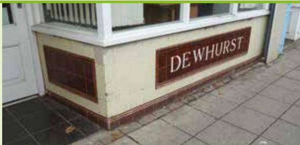
A tiled stallriser on a former butchers shop. Tiles provide an attractive decorative feature but can be vulnerable to knocks, especially on the corners. Internal bathroom type tiles are not acceptable in appearance and would not be suitable for outdoor use.
