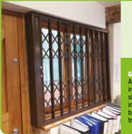
**GOOD DESIGN.** An example of an internally fitted horizontal sliding shutter as used in some timber framed buildings without traditional shopfronts.
