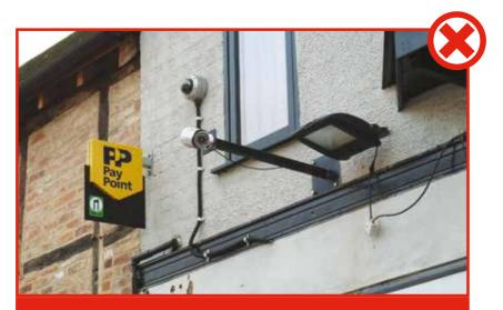
**POOR DESIGN.** Poorly located CCTV cameras with prominent wiring on a front elevation, it is unlikely that both are necessary in this location and one should be removed.
