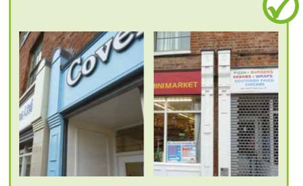
**GOOD DESIGN.** An open security shutter with the shutter box hidden behind the facia and the side runners hidden inside the pilaster. *Above right.* The pilasters showing the shutters open and in closed positions.
