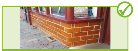
A glazed brick stallriser with a wooden cill above. Glazed bricks are easy to source and provide a robust and attractive shopfront feature.
