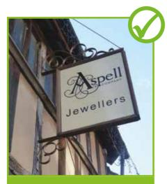
**GOOD DESIGN.** A well-designed projecting sign on an attractive wrought iron bracket in Spon Street. The sign has been carefully located to respect the appearance of the building and fits tidily on to a stud in the timber frame.
