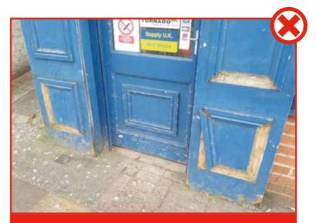
**POOR DESIGN.** Tacked-on moulding has been used to create decorative panels on this shopfront but they are poor quality, vulnerable to damage and quickly look tatty. Proper joinery techniques need to be used on timber shopfronts if they are to be robust and attractive.
