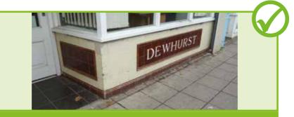
A tiled stallriser on a former butchers shop. Tiles provide an attractive decorative feature but can be vulnerable to knocks, especially on the corners. Internal bathroom type tiles are not acceptable in appearance and would not be suitable for outdoor use.
