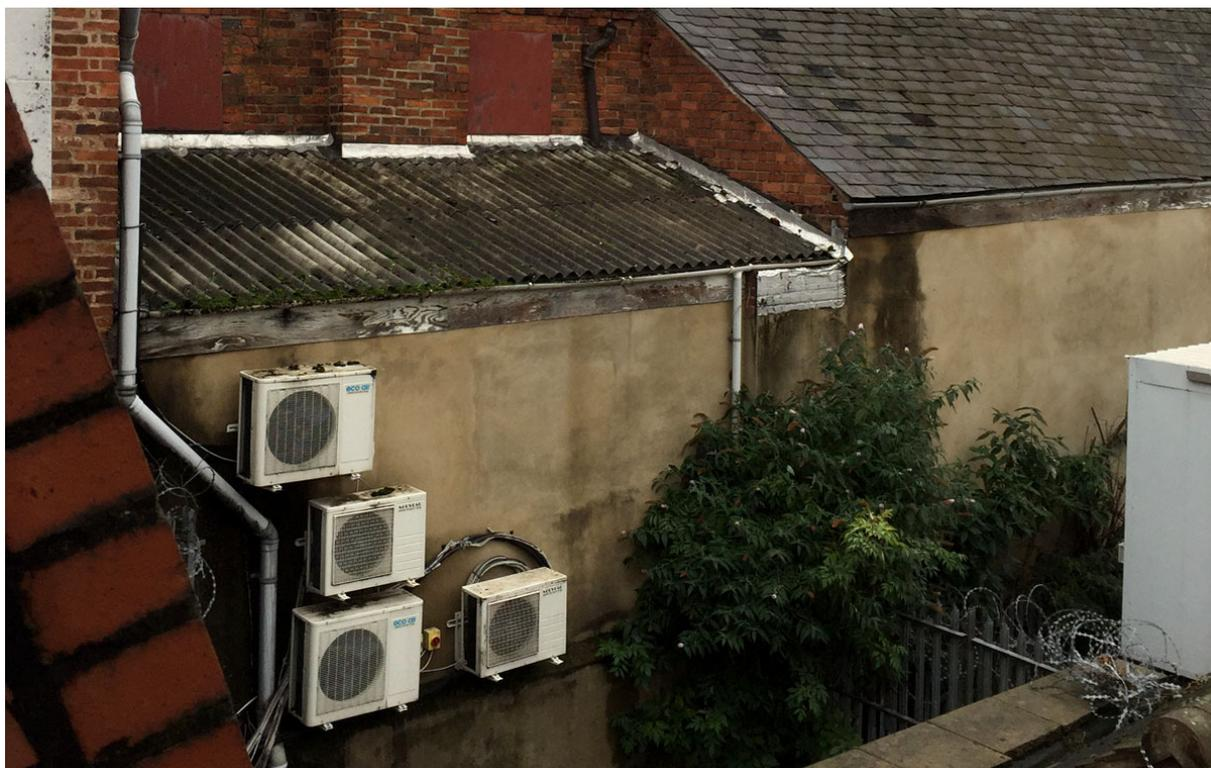
Figure 71. Burges rear view. Note windows blocked with sheet steel, uPVC rainwater goods, corrugated sheet roofing, a/c condensers, steel security fencing, razor-wire, and vegetation
