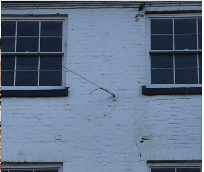
4. Facade to No. 31 Cross Cheaping - note cracks in facade and infill brickwork to spandrel panels above first floor windows
