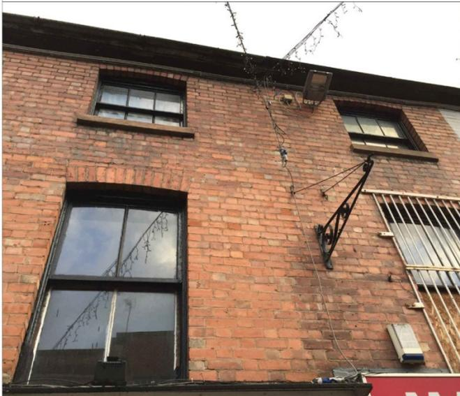
3. Facade to No.'s 28 & 29 Burges illustrating typical brickwork and variation in window types and condition
