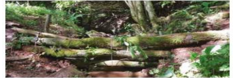
A series of 24 woody dams installed in Cumrew beck to reduce flooding in Cumrew village, near Carlisle. © Eden Rivers Trust
