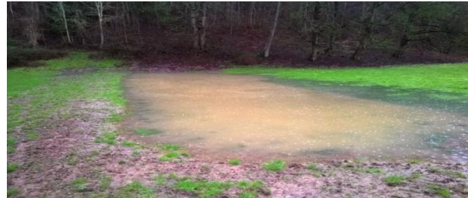
Swale to divert and hold surface runoff © Eden Rivers Trust
