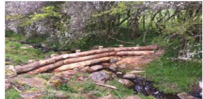
Leaky barriers on Dovenby beck, near Cockermouth © West Cumbria Rivers Trust
