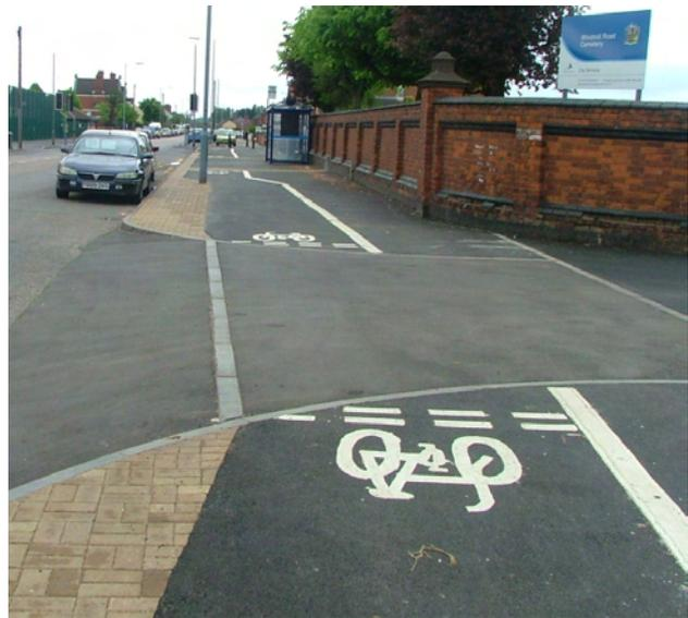
Cycle track with block paving buffer strip
