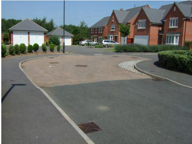
**Speed control bend with contrasting paving
