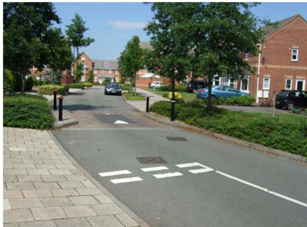
**Give way narrowing as a speed restraint measure**
