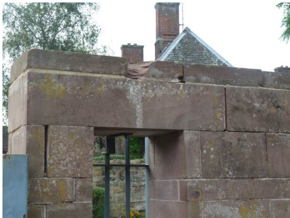
Damage to sandstone wall
