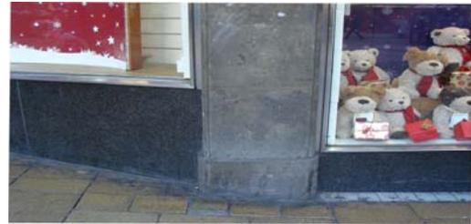
Figure 35: Materials: Granite, Horton stone & stainless steel
