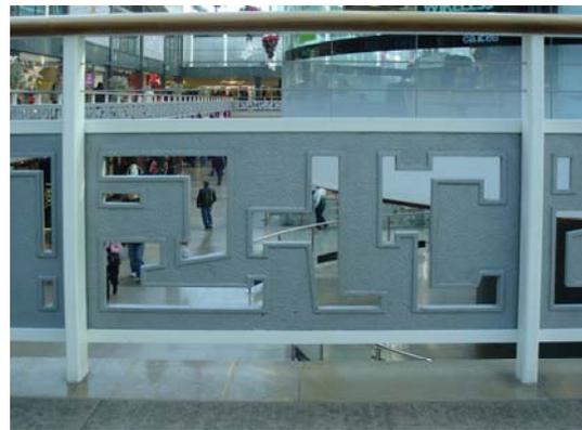
Figure 42: Cast aluminium balustrade
