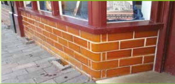
A glazed brick stallriser with a wooden cill above. Glazed bricks are easy to source and provide a robust and attractive shopfront feature.
