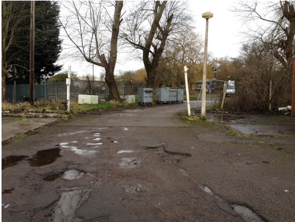
Figure 2.3: Photograph 2 – Blocked highway drains running through the site.
