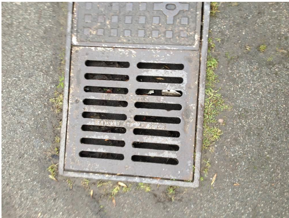
Figure 2.3: Photograph 2 – Blocked highway drains running through the site.
