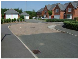
Speed control bend with contrasting paving and override area
