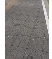
**Charcoal Tactile –** for crossing points. They provide a suitable contrast to light paving. Not suitable for tarmac foot paths.
