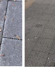
Charcoal Tactile – for crossing points. They provide a suitable contrast to light paving. Not suitable for tarmac foot paths.
