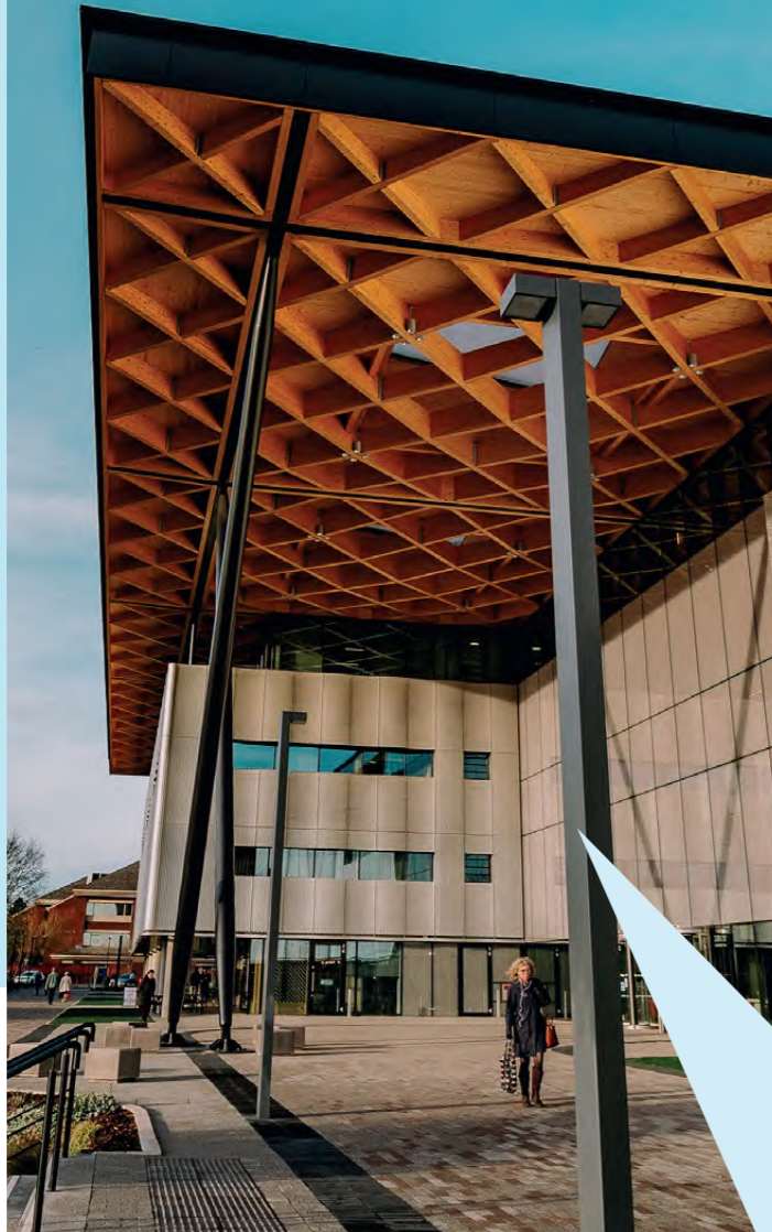
Lord Bhattacharyya Building, University of Warwick, home of the National Automotive Innovation Centre and RIBA National Award Winner 2021
