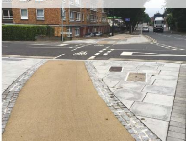
Figure 10.14: Full set back, marked priority (bent-out) crossing, Enfield
